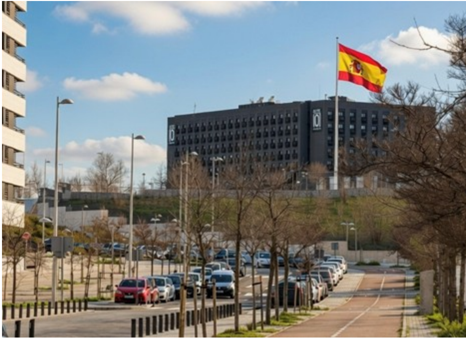
(Actual photo of the 680-room Hotel101 in Madrid, Spain)
