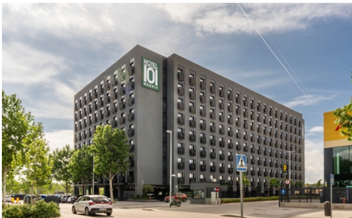
Latest Photo of 680-room Hotel101-Madrid
